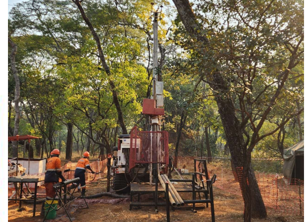
Drilling is underway at Mumbeszi
