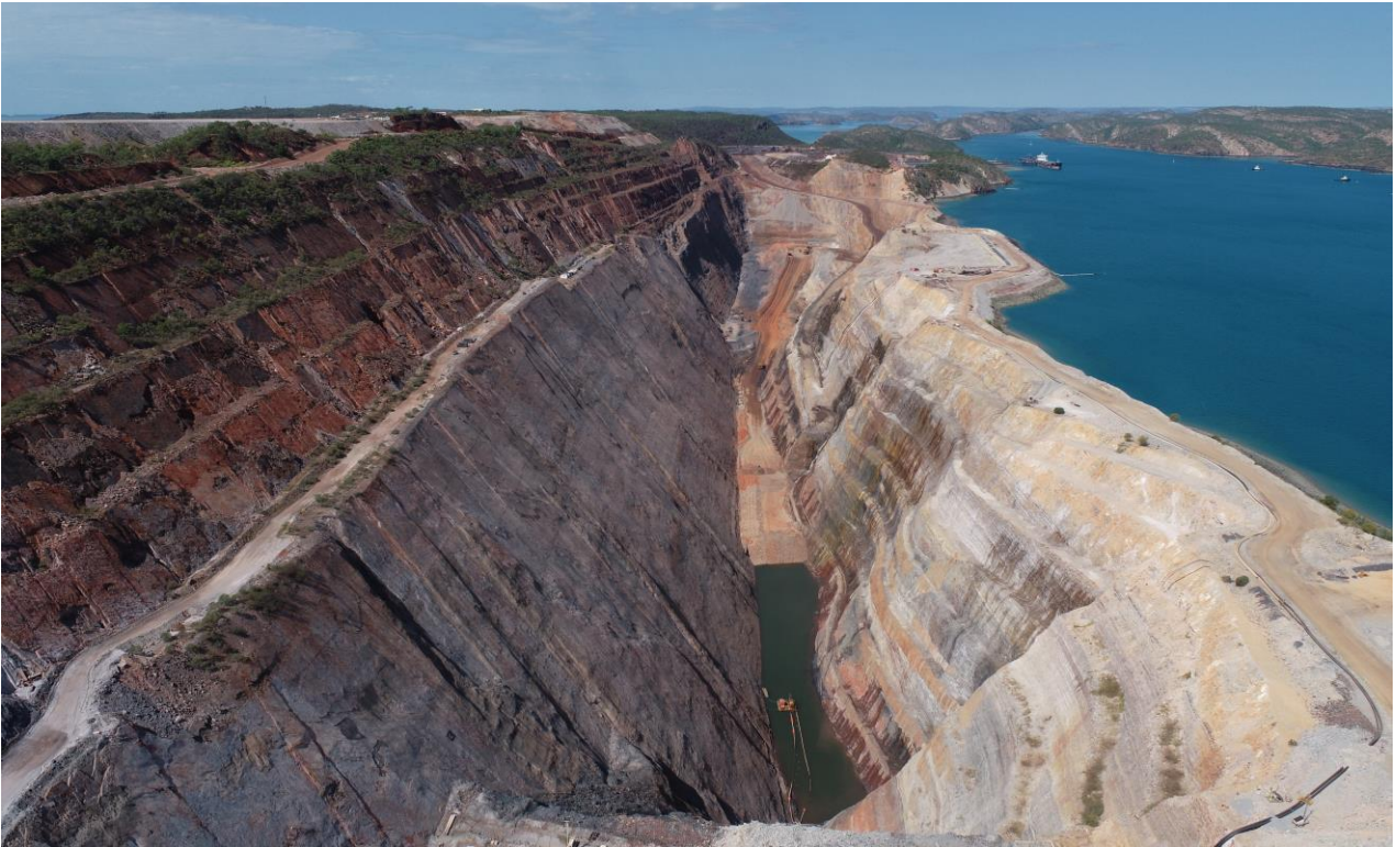
Figure 1: Koolan Island Main pit, looking to the east over the completed western end showing haul ramp-repositioning and switchback construction work and the western water management sump, July 2024.
