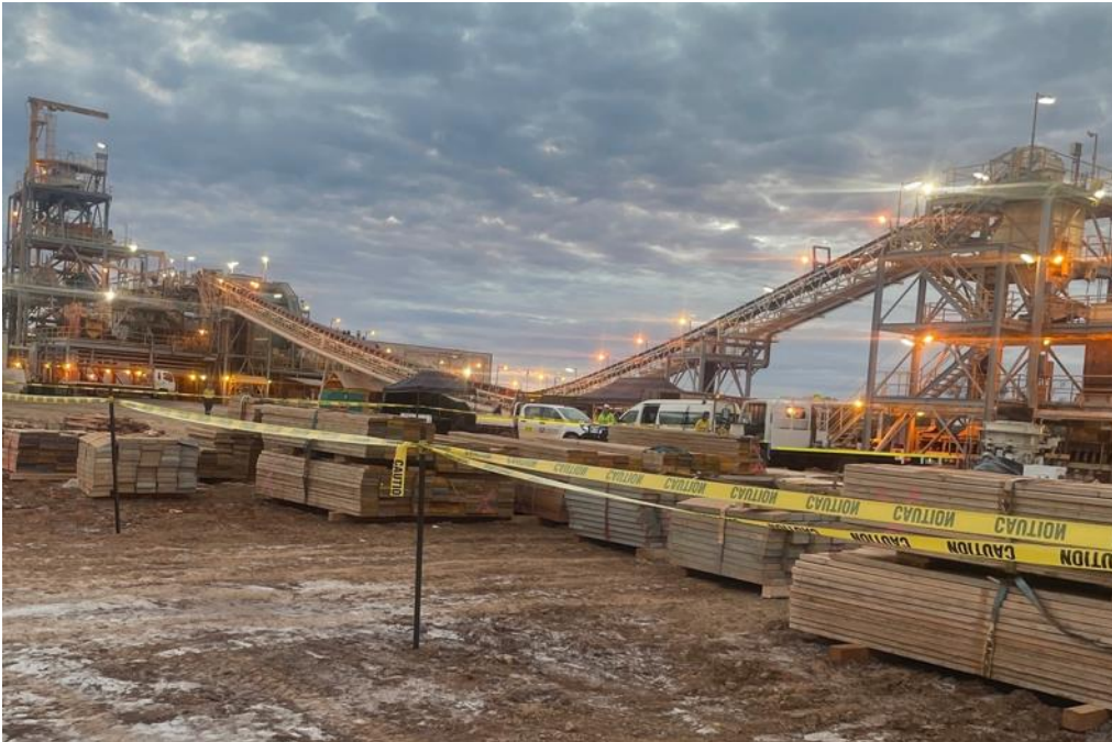
Figure 6. Laverton mill re-start - Scaffolding delivered
