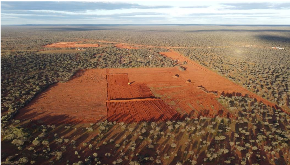
Figure 7. Hub open pit - Clearing site
