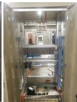
MCC CABINET CENTRE & ONE WITH DOOR OPEN
