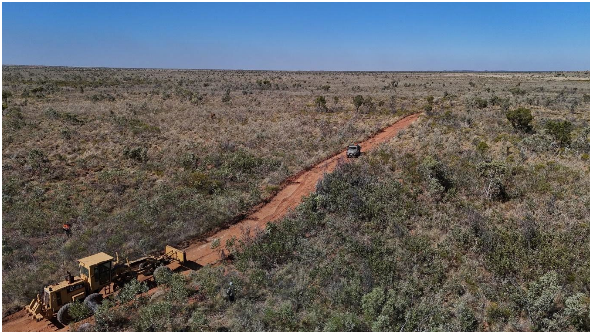
Image 1: Earthmoving underway at Trek’s Christmas Creek Project.
