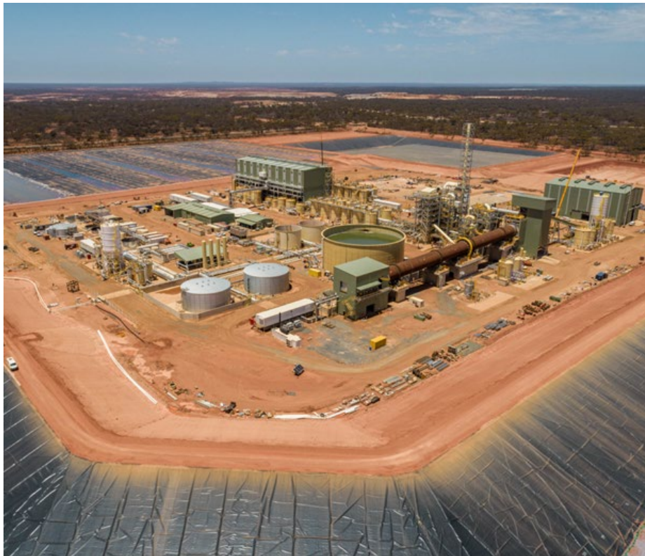
Lynas Kalgoorlie Rare Earths Processing Facility
