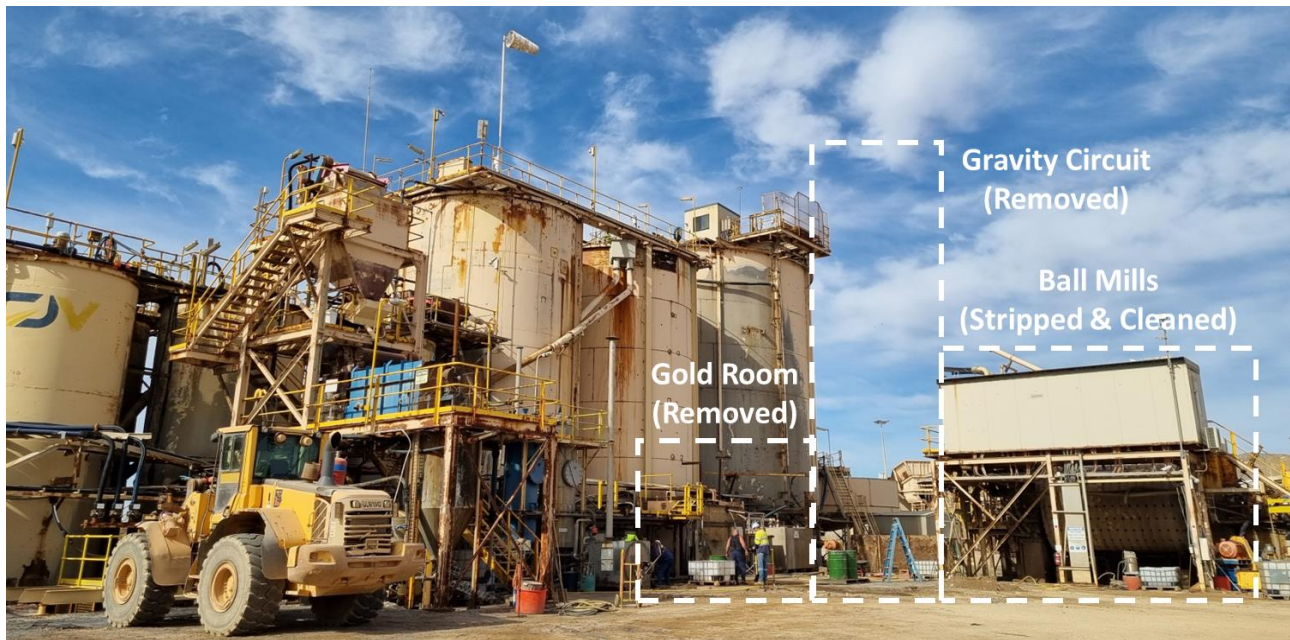
Fig 5 – Central Gawler Mill with gravity circuit, gold room and other key equipment removed 11
