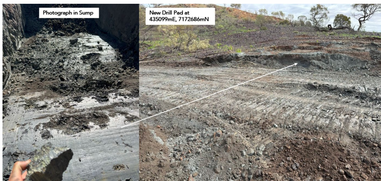
Figure 2: Graphitic material intersected during RC pad preparation earthworks at Graphite Bull, July 2024.
