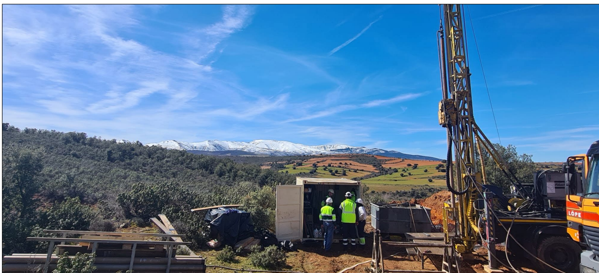
Figures 2: Drill rig commencing drilling at the Iberian One Project, Spain March 2024.
