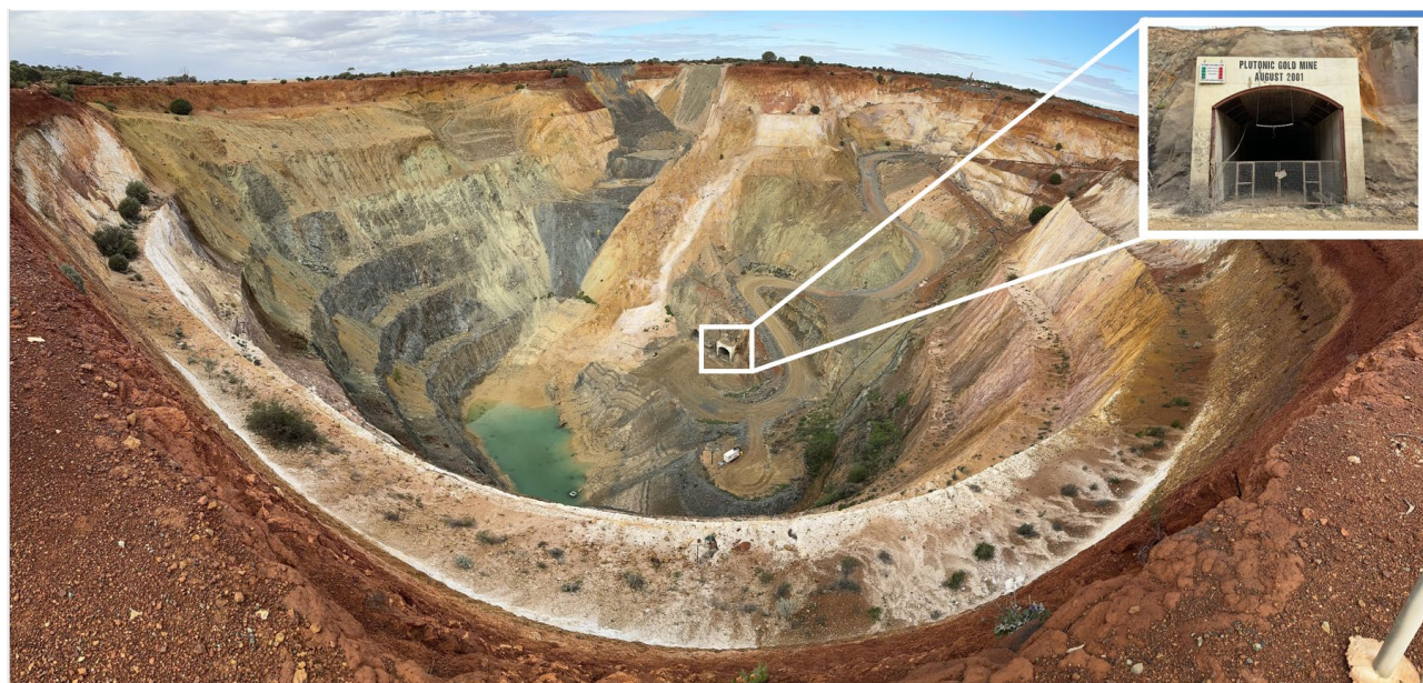
Figure 6: Plutonic East open pit and underground portal – dewatering progress
