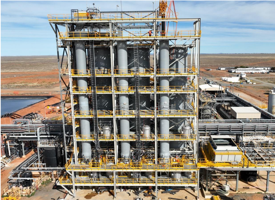
Figure 1: Construction of NIMCIX columns 2 and 3 nearing completion
