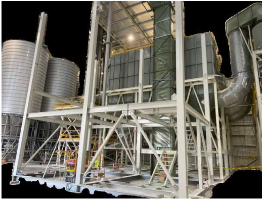
Figure 1: Classifier Structure progress with Bucket Elevator installed at rear
