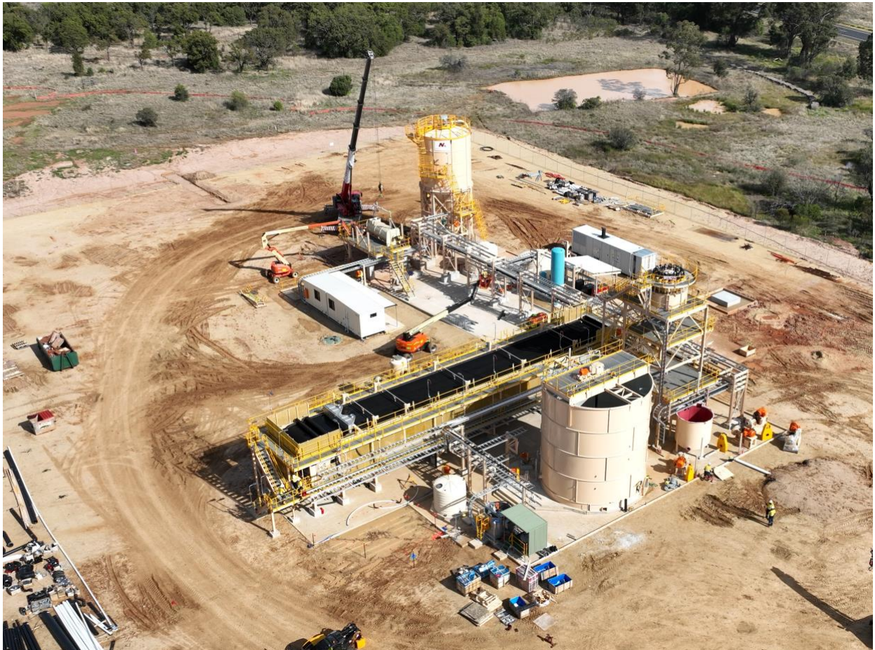
Paste plant structural works
