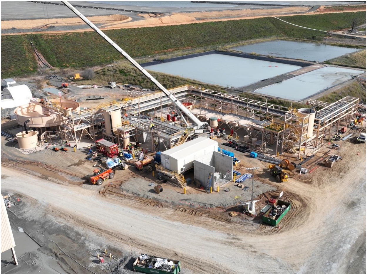
Process flotation and fine grind circuit structural works
