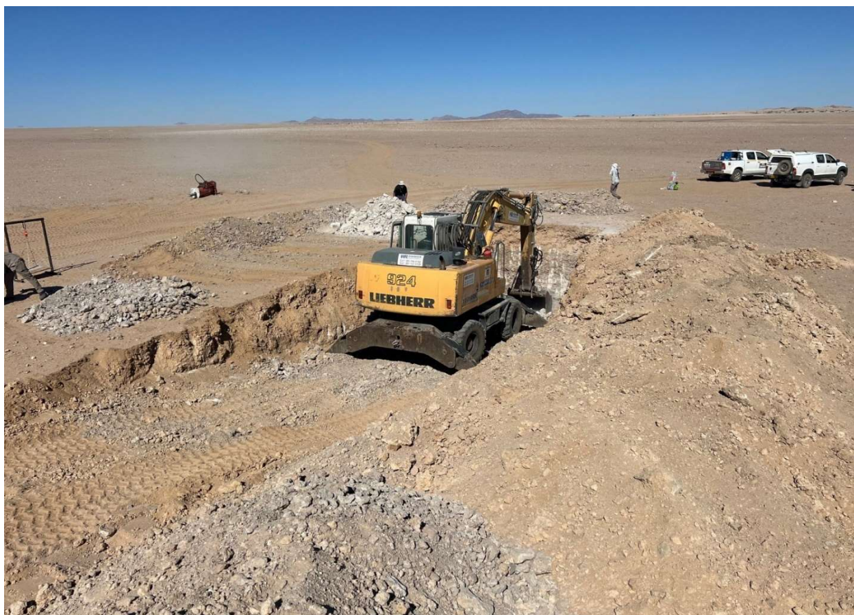
Figure 5 First Test Pit Excavated at Koppies
