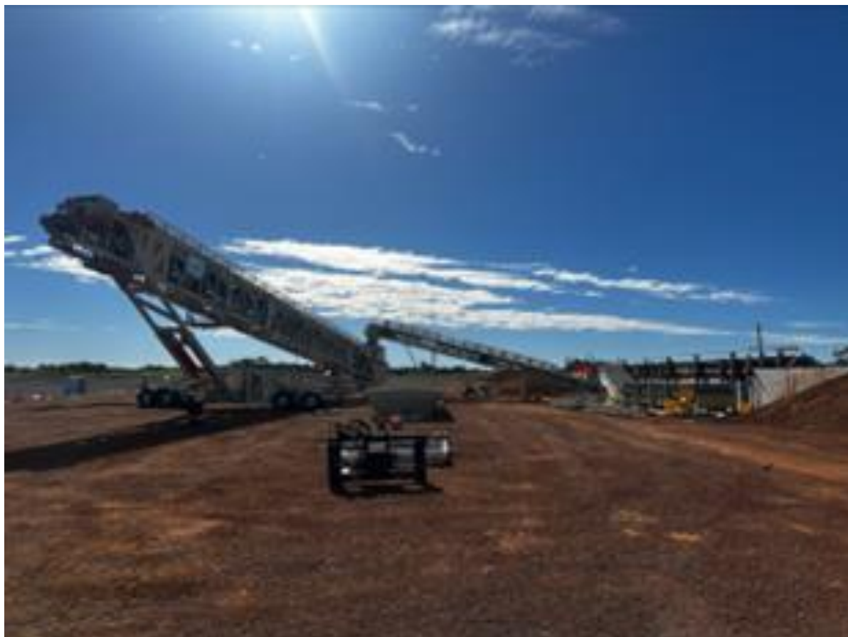
Ruvidini Inland Port Construction – July 2024
