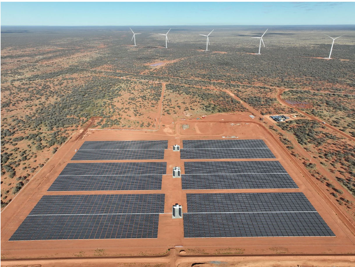
Figure 20: Aerial view of solar farm and wind turbines
