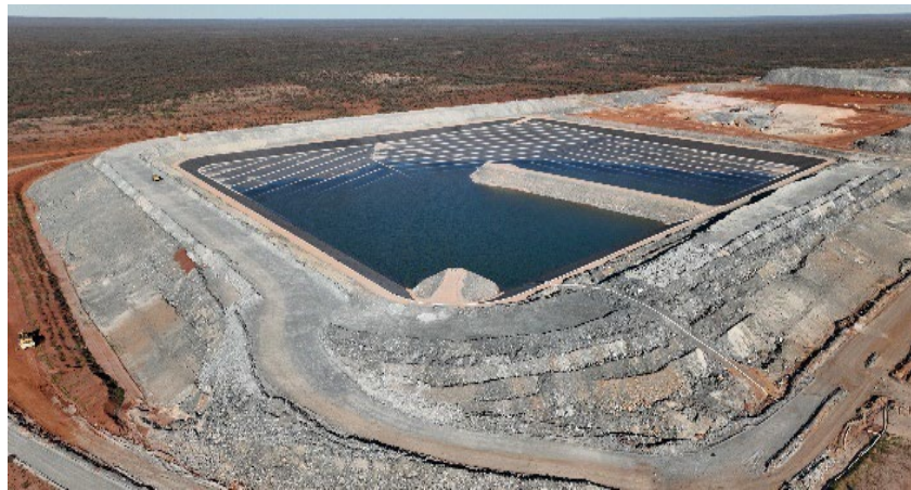
Figure 9: Tailings Storage Facility (TSF) Cell 1
