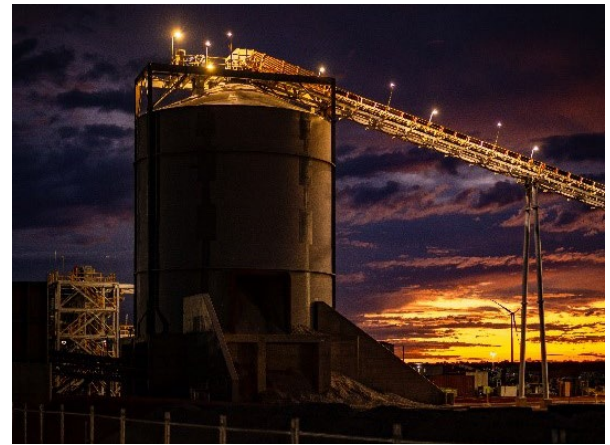
Figure 11: 4000t Fine Ore Bin – filled to capacity
