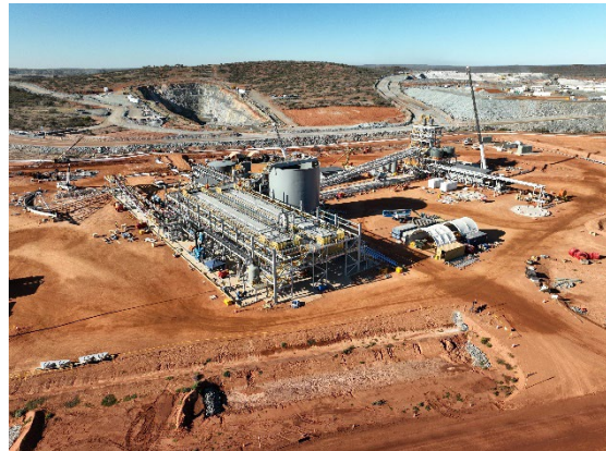
Figure 8: Paste Fill Plant construction well underway
