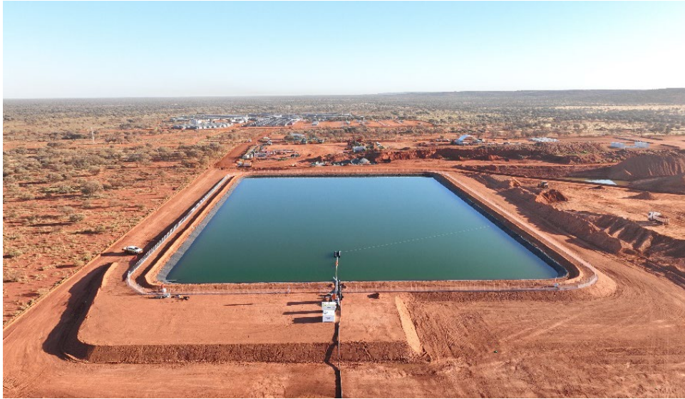
Figure 21: Supplementary Raw water storage dam
