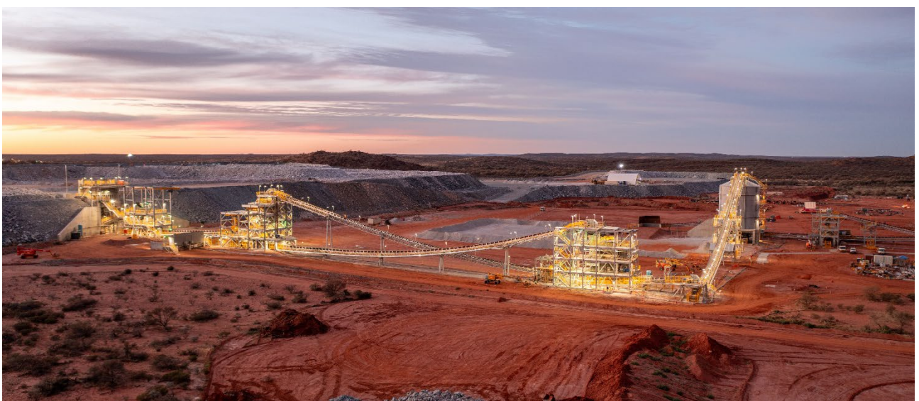
Figure 14: Side view of Crushing Plant
