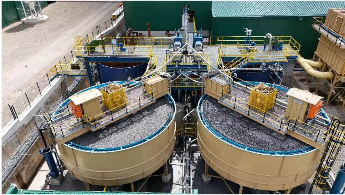
Figure 4: Vares Processing Plant
