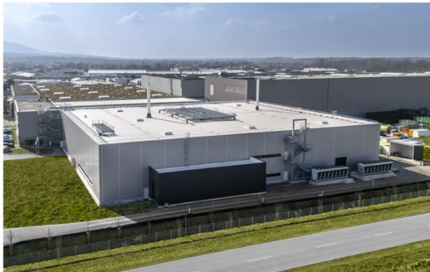
Figure 4 – Mercedes-Benz LiB Recycling Building, Kuppenheim Germany.
