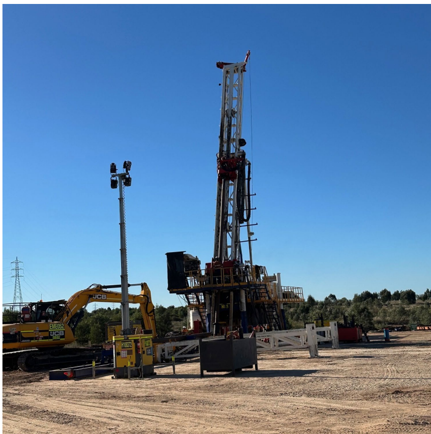
Figure: Lucas rig drilling second lateral
