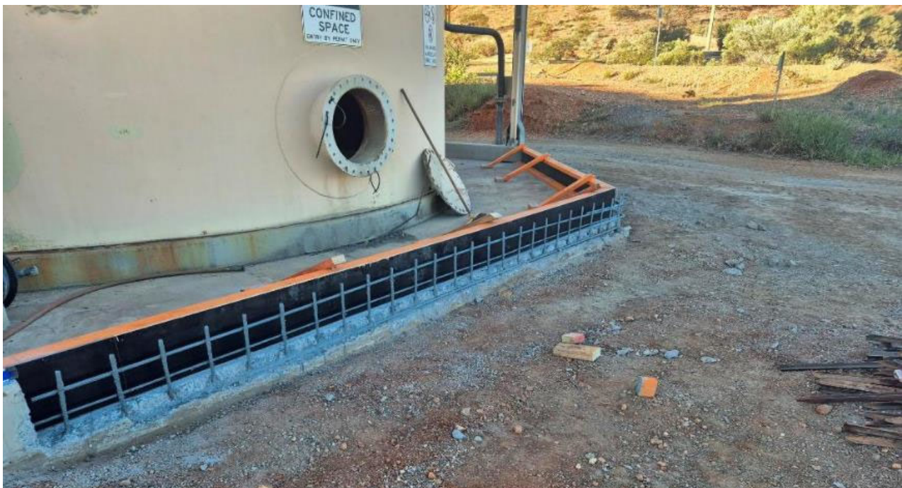
Figure 10: Remedial concrete works
