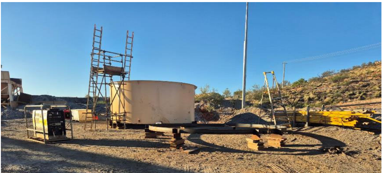
Figure 6: New CIL top of tank ring ready for installation
