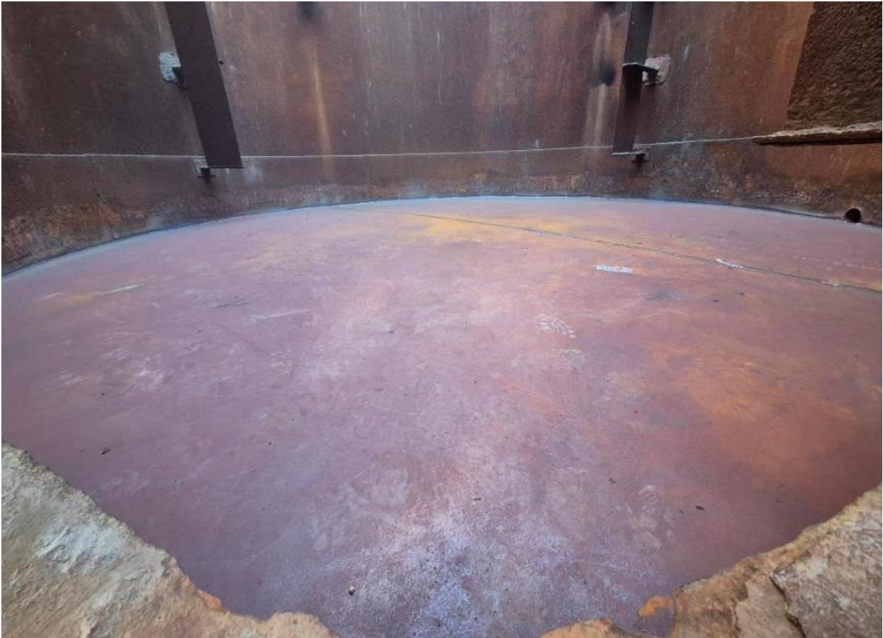
Figure 5: CIL tank floor repairs underway
