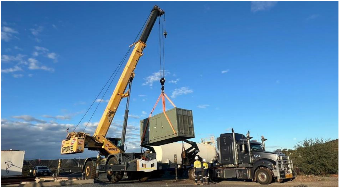
Figure 1: Power station #2 generator installation
