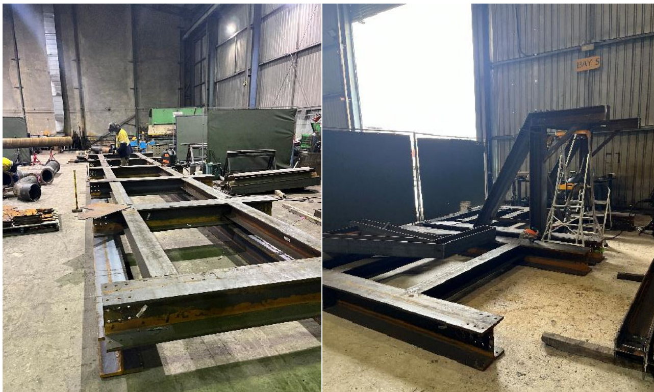
Figure 2: ROM wall fabrication progressing to plan
