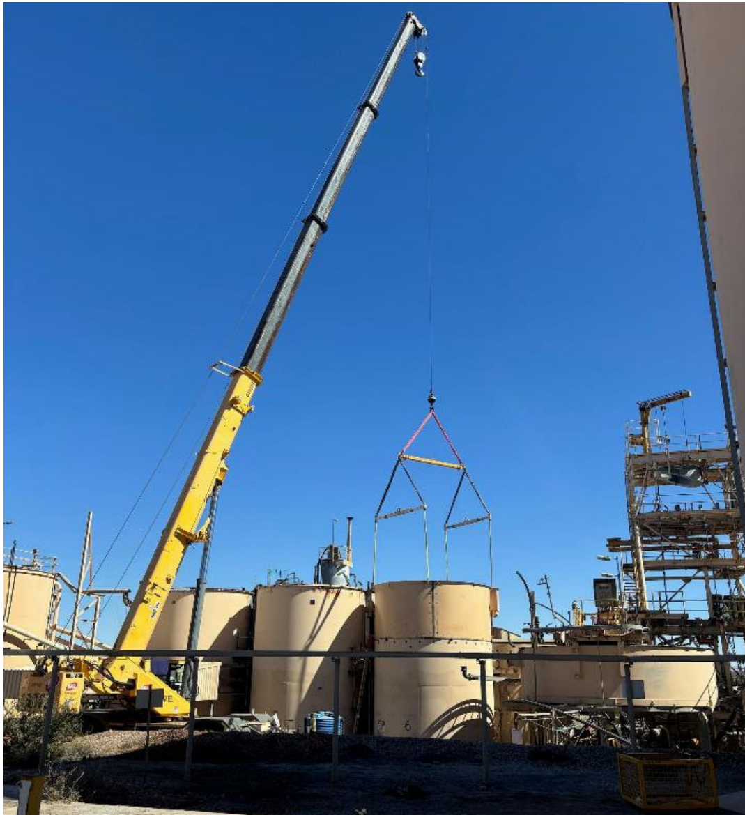
Figure 7: First CIL tank rings to be installed
