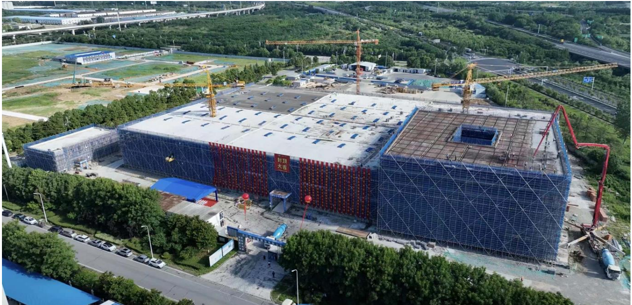
Photo: Vmoto's new manufacturing facilities in Nanjing, China under construction
