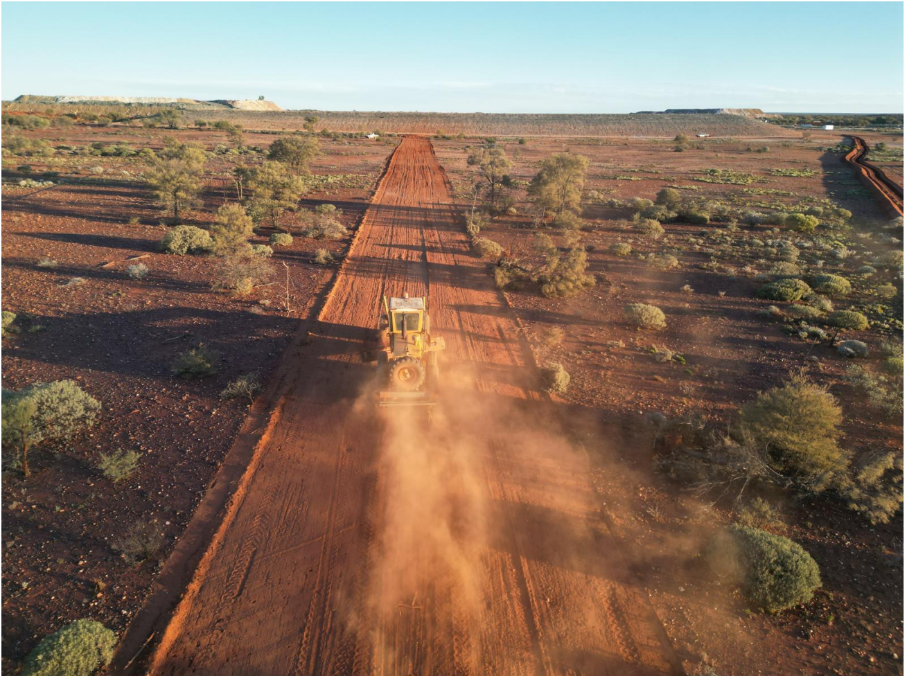
Figure 1: Haul road construction underway, July 2024.
