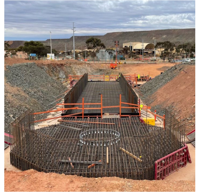
Flotation Thickener Concrete Works
