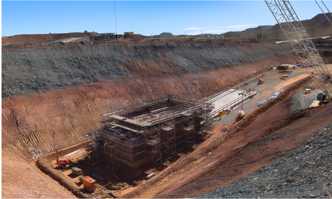
Primary Crushing Area Concrete Works
