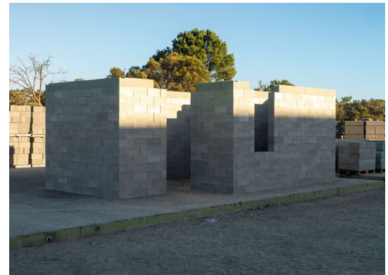
Outdoor SAT-style build completed prior to Hadrian X ® leaving Perth
