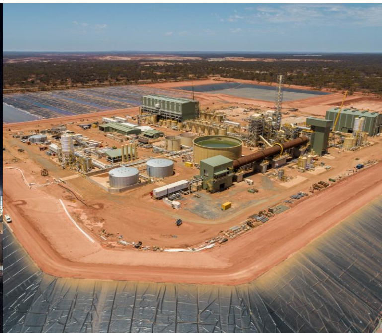
New Kalgoorlie Rare Earths Processing Facility
