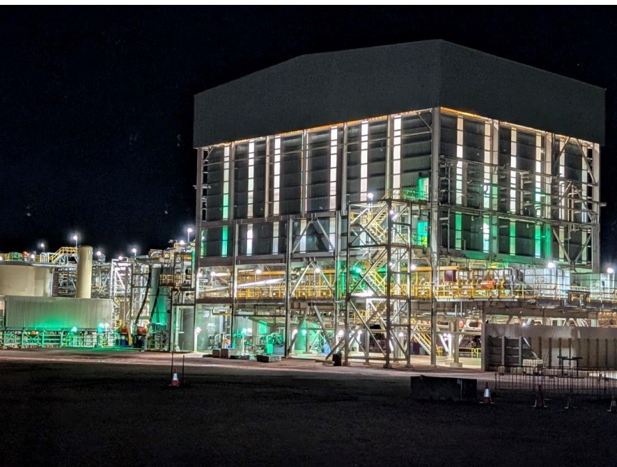
Mt Weld Expansion
