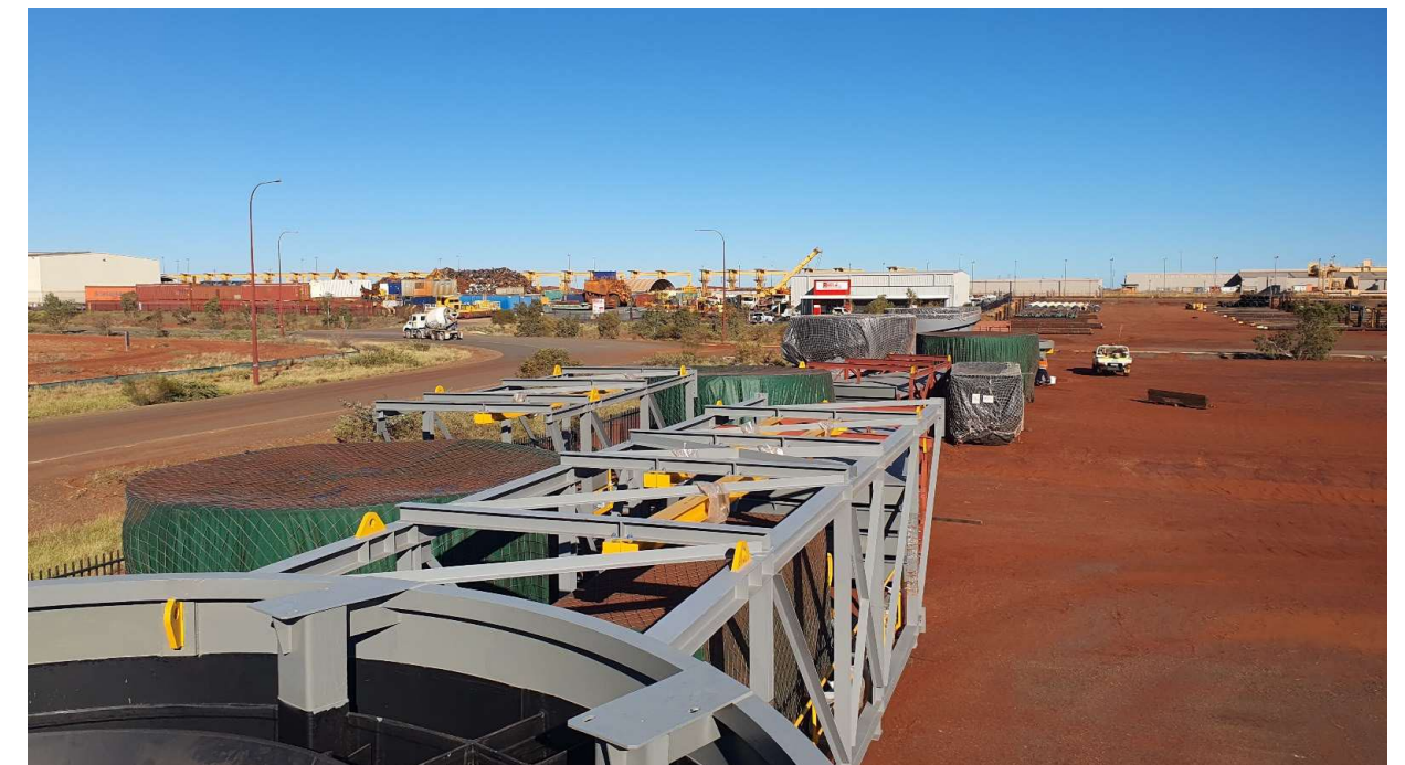
Flotation Cells & Structural Steel ready for installation.
