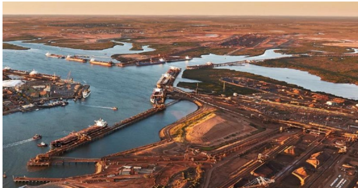
Utah Point Facility and regional infrastructure.
