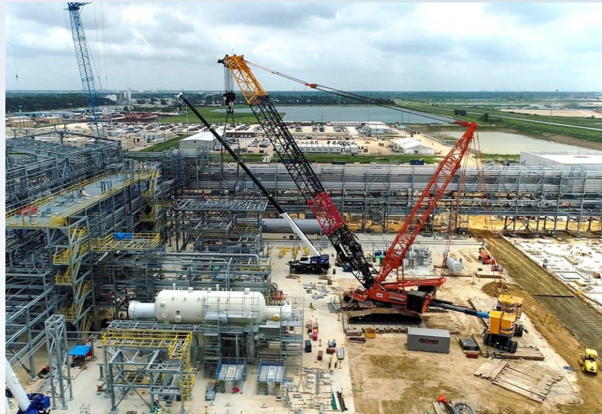
Construction of OCI's Clean Ammonia Project
