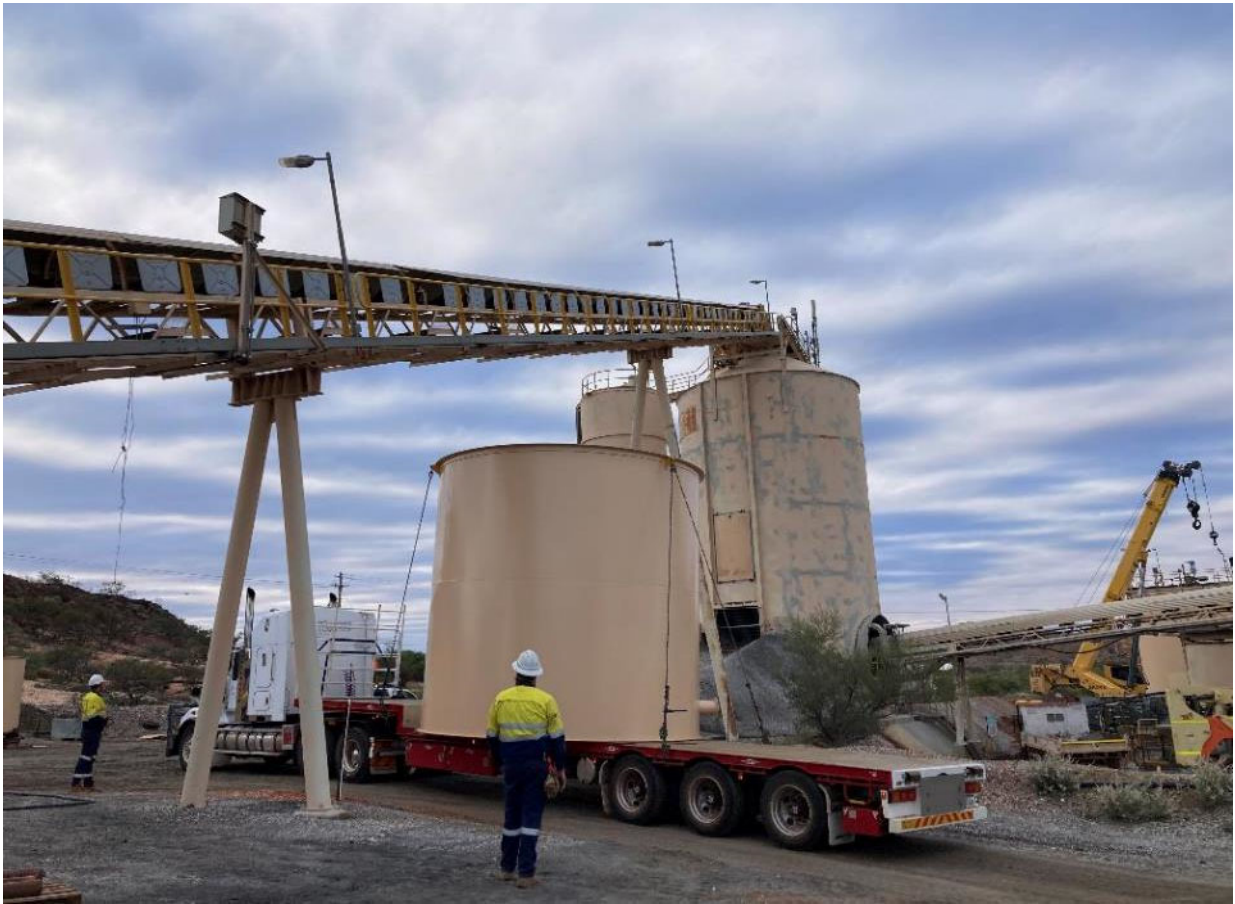
Figure 7: Process water tank arriving.
