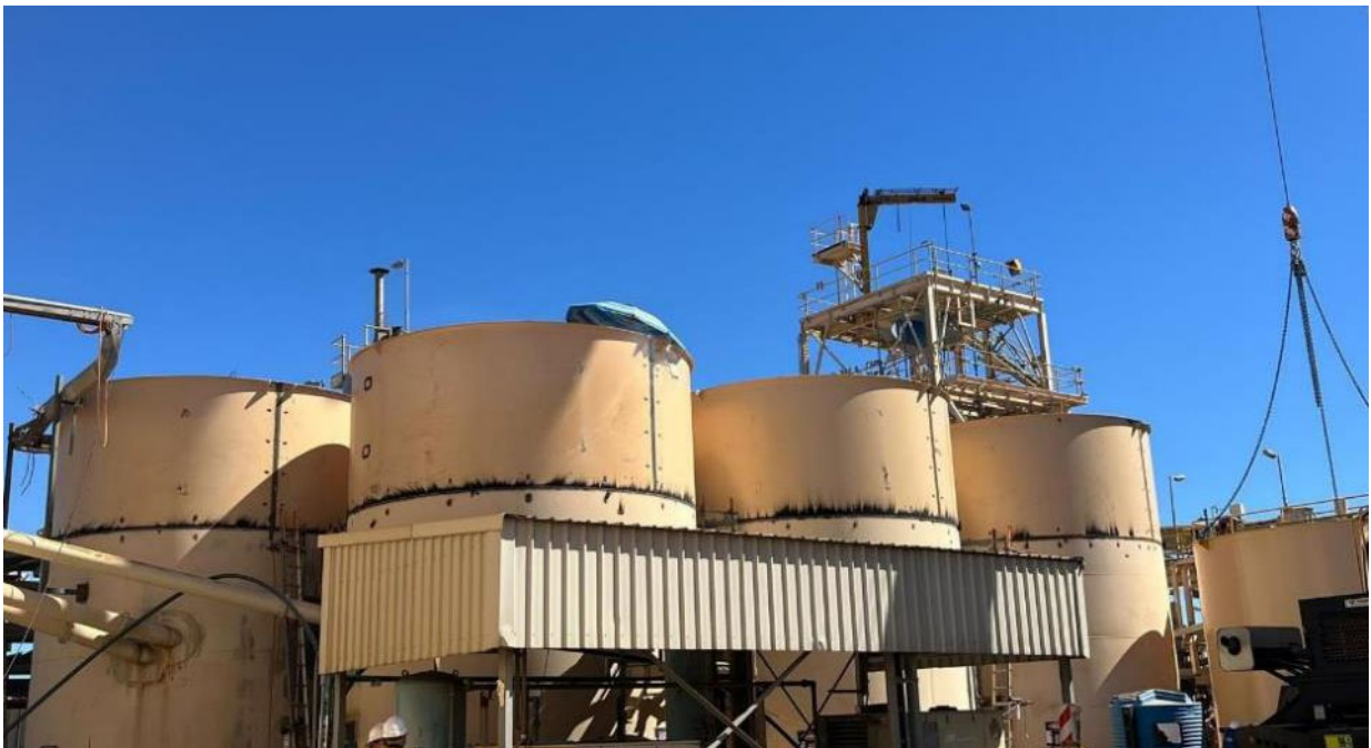
Figure 8: Top rings on CIL tanks all in place and process water tank being installed.
