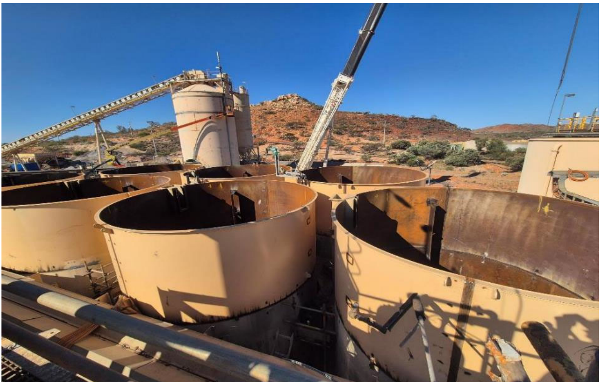
Figure 6: All CIL top of tank strakes installed.
