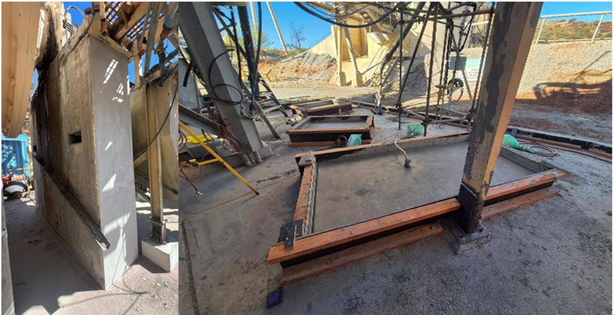
Figure 10: Remedial concrete works completed including the mill plinths and pump bases.
