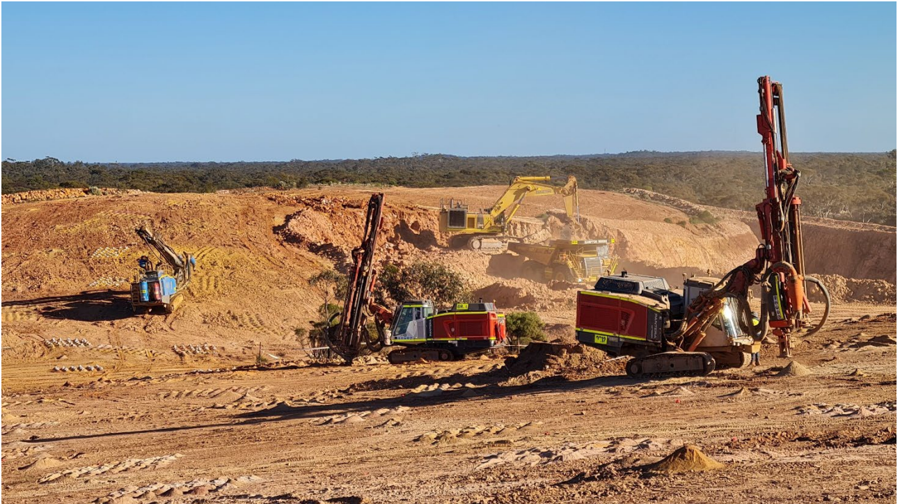
Figure 4: Drilling second shot with load and haul operations in background (27 August 2024)
