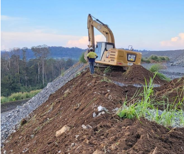
Figure 19 | Okvau batter/berm trial
