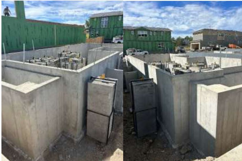
Figures 1 & 2 First EdenCrete® Pz7 project- Foundation walls for home development – Colorado
