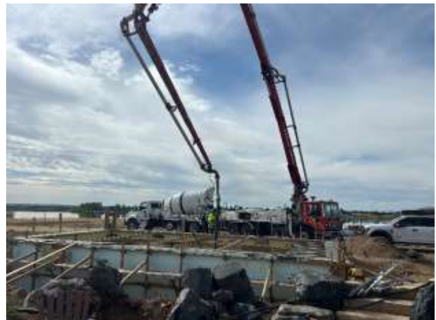
Figures 7 & 8 - Colorado swimming pool contractors utilizing EdenCrete for crack reduction
