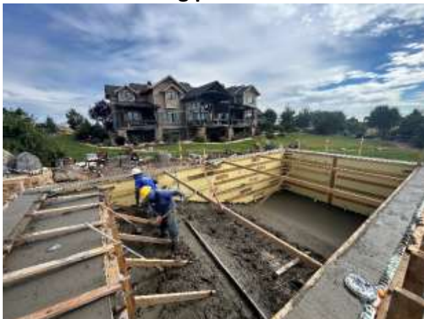
Figures 7 & 8 - Colorado swimming pool contractors utilizing EdenCrete for crack reduction
