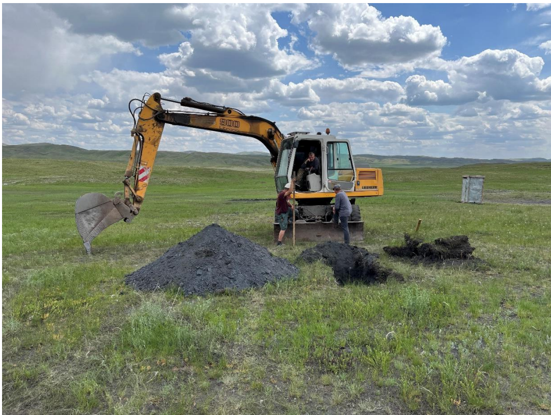
Figure 1 - Test Pitting at Sarytogan in 2022. Similar sized excavator to be used for 20t trial mine this week.
