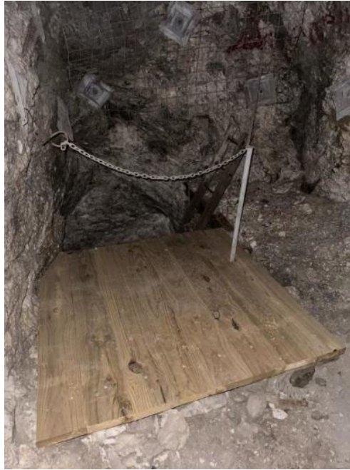
Figure 5: One of the rehabilitated escapeway platforms being installed throughout the mine.
