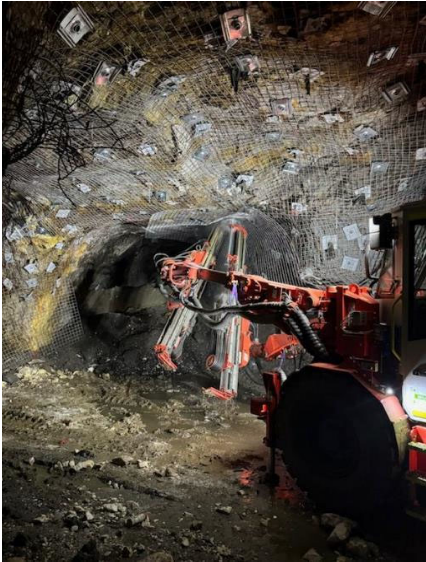
Figure 8: Twin boom Jumbo conducting ground support rehabilitation in the 1007 Level access to open up multiple high-grade drives.
