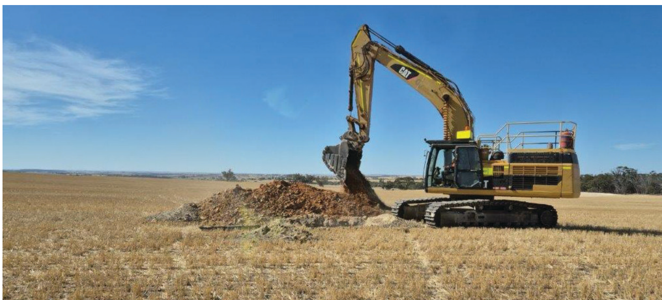
Figure 10 – Excavator digging a geotechnical test pit beneath the planned Tailings Storage Facility
