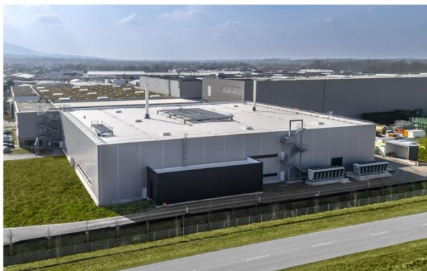
Figure 4 – Mercedes-Benz LiB Recycling Building, Kuppenheim Germany.
