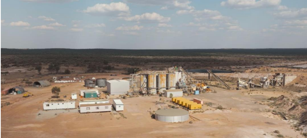
Figure 17 - Brightstar Processing Plant looking southeast
