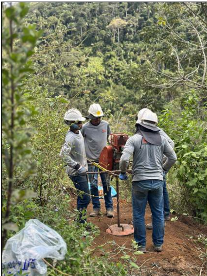
Figure 5: EQN Auger Drilling Team at Campo Grande
