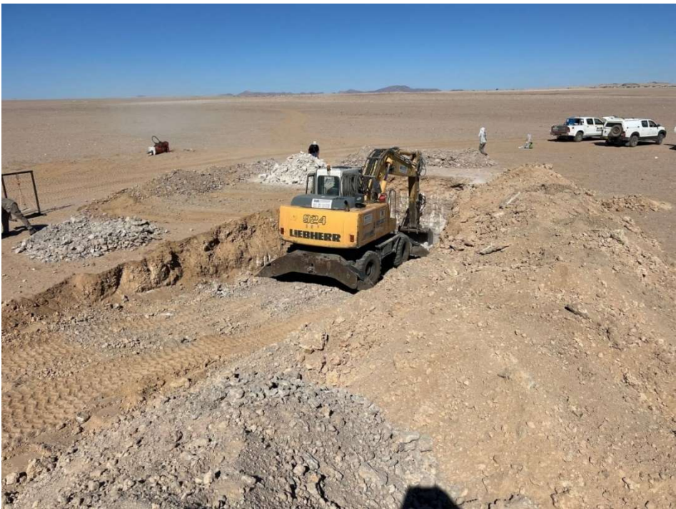
Figure 5 – Test Pit Excavation at Koppies Resource
