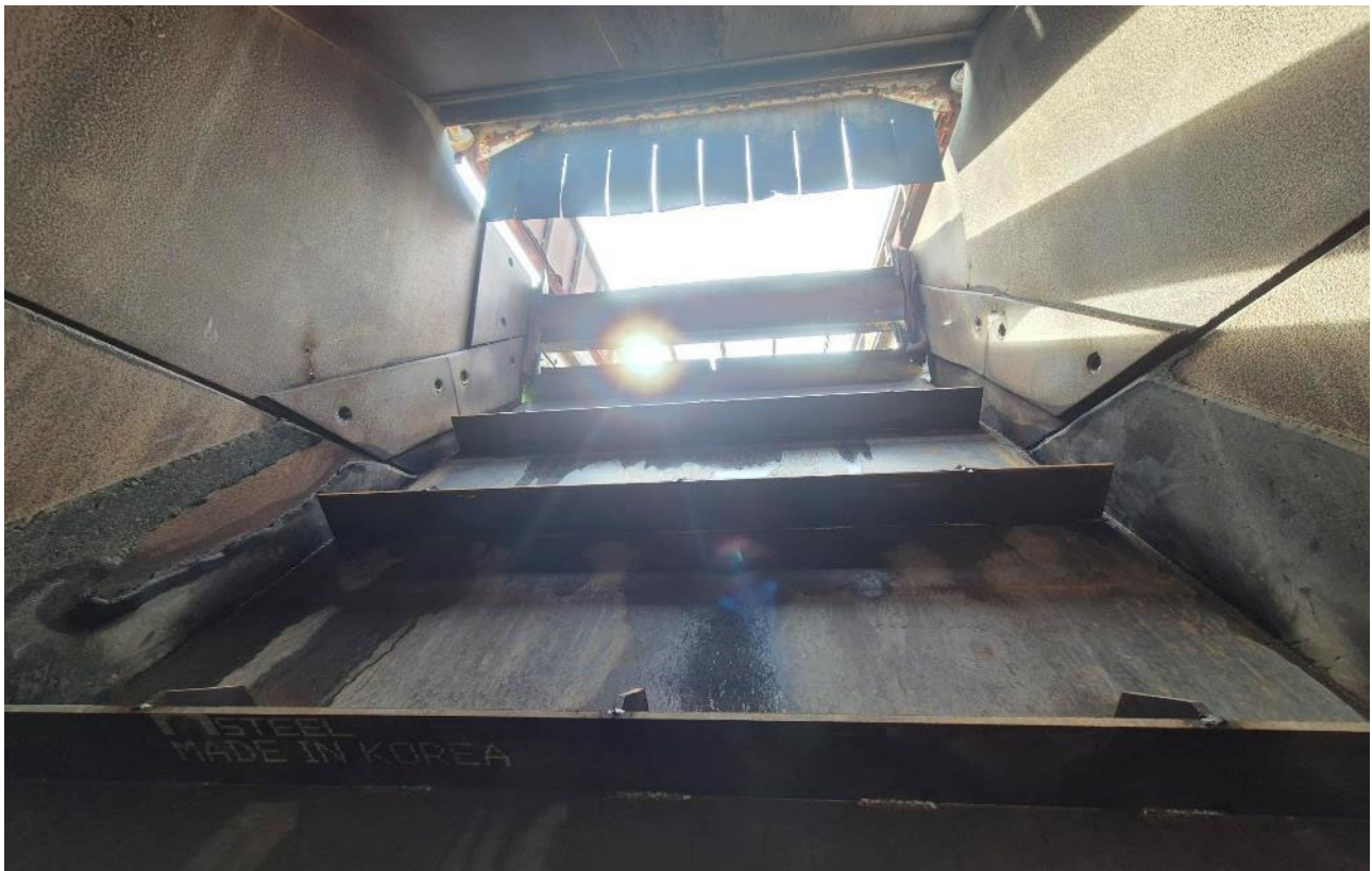
Figure 4: Screen deck rock ledge repairs completed.
