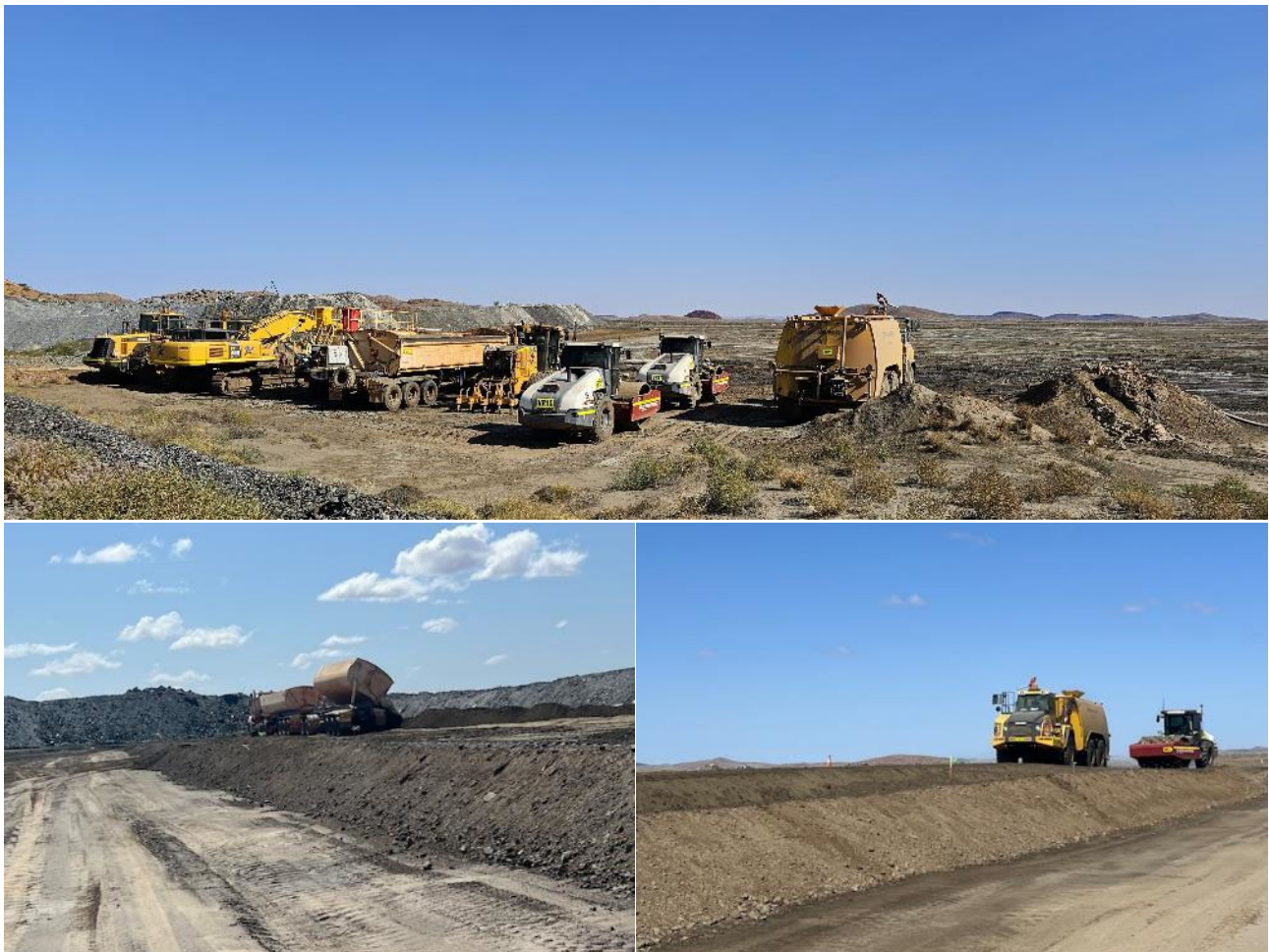
Figure 13: TSF works underway and will be ready for December 2024 commissioning.
