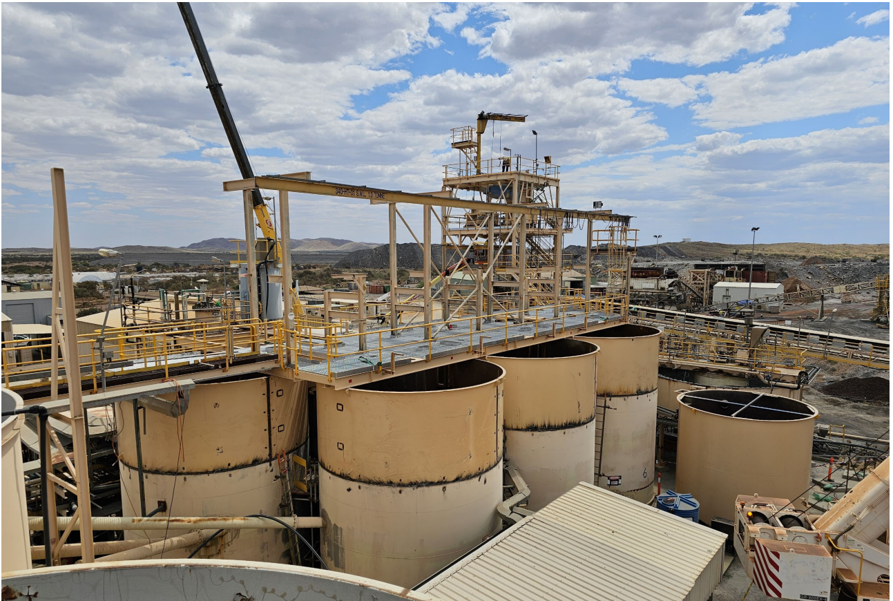
Figure 5: Top of tank structure completed and walkways ~80% complete.
