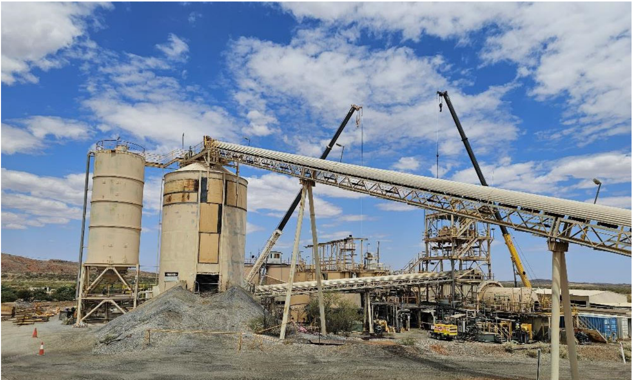
Figure 1: Paulsens processing facility refurbishment is on track for December 2024 commissioning. Conveyor CV11 feeding the fully repaired fine ore bin.
