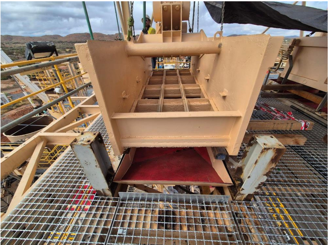
Figure 10: Gravity screens and underpan installation.
