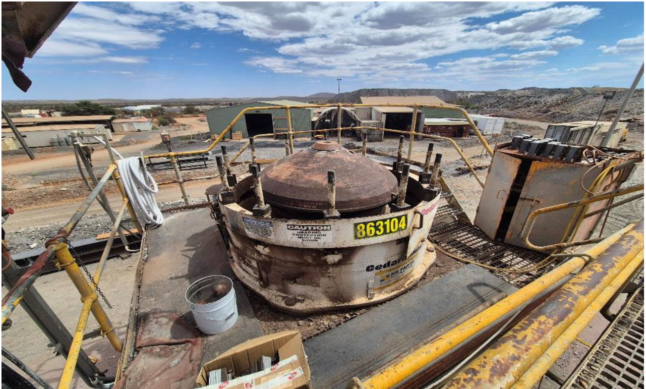
Figure 3: Cone crusher repairs completed.
