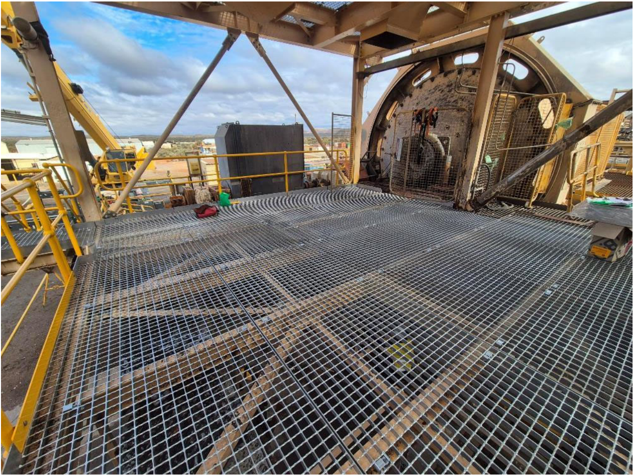
Figure 7: Mill deck grid mesh replacement completed.
