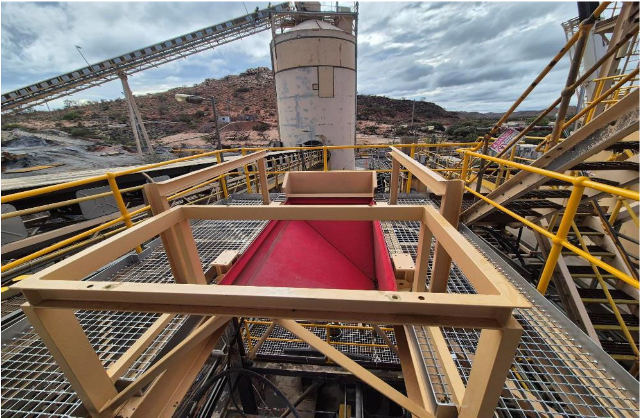
Figure 9: Trash screen deck completed and underpan installed.
