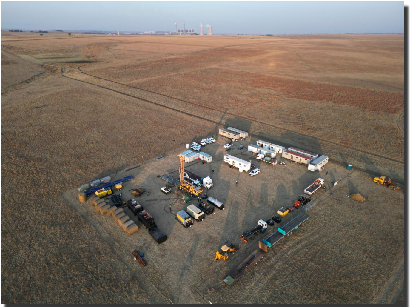
Figure 2 shows the production drilling rig on site for spudding well 271-23PT with Majuba power station in the background.
