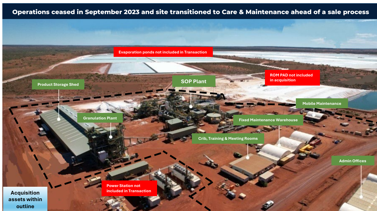
Figure 1 – Photograph of the Beyondie Potash Project in 2023 when operated by Kalium. The Transaction comprises a fully constructed processing plant, site offices and maintenance infrastructure. Specific plant components include, KTMS crushing circuit, Kainite conversion circuit, column flotation circuit, liquor cooling heat exchangers, evaporative cooling circuit, product separation centrifuges, SOP recovery and granulation units, RO water plant and a bulk storage shed.
