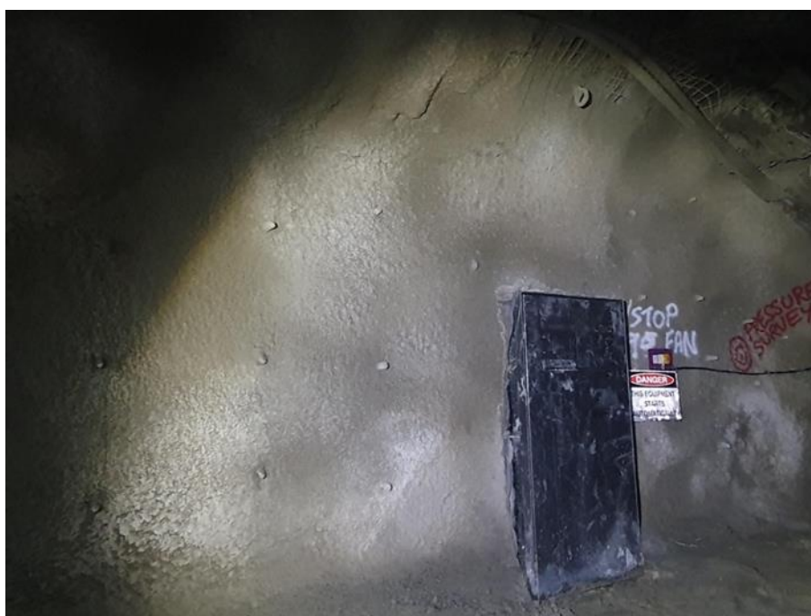
Figure 5: Vent door closing off ventilation recirculation, set in shotcrete and cable bolts for additional ground support.
