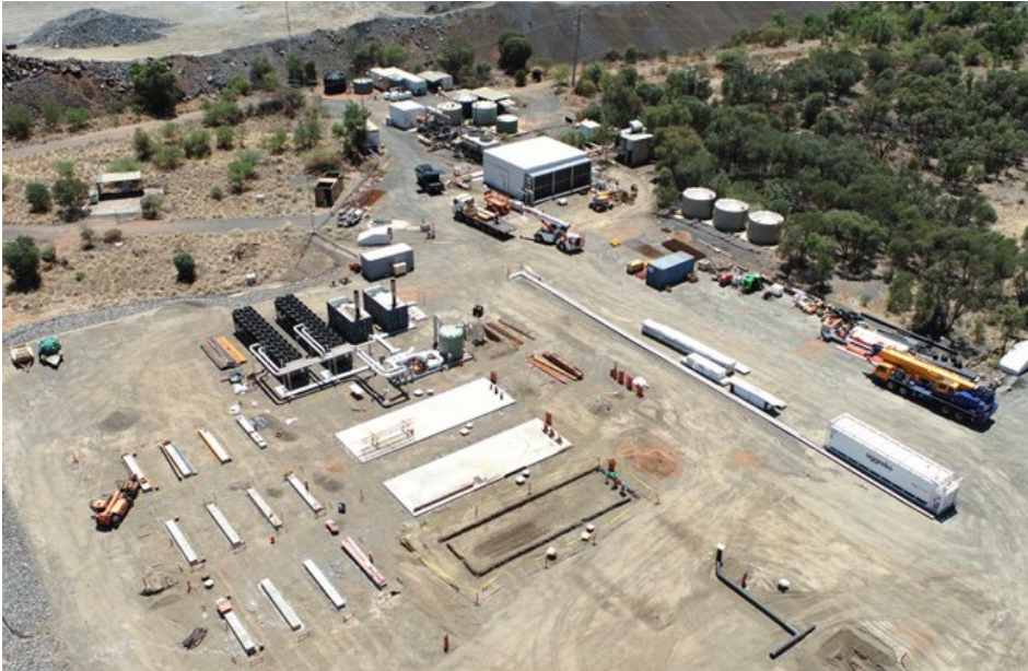
Photo 1. New mine ventilation cooling system – construction work
