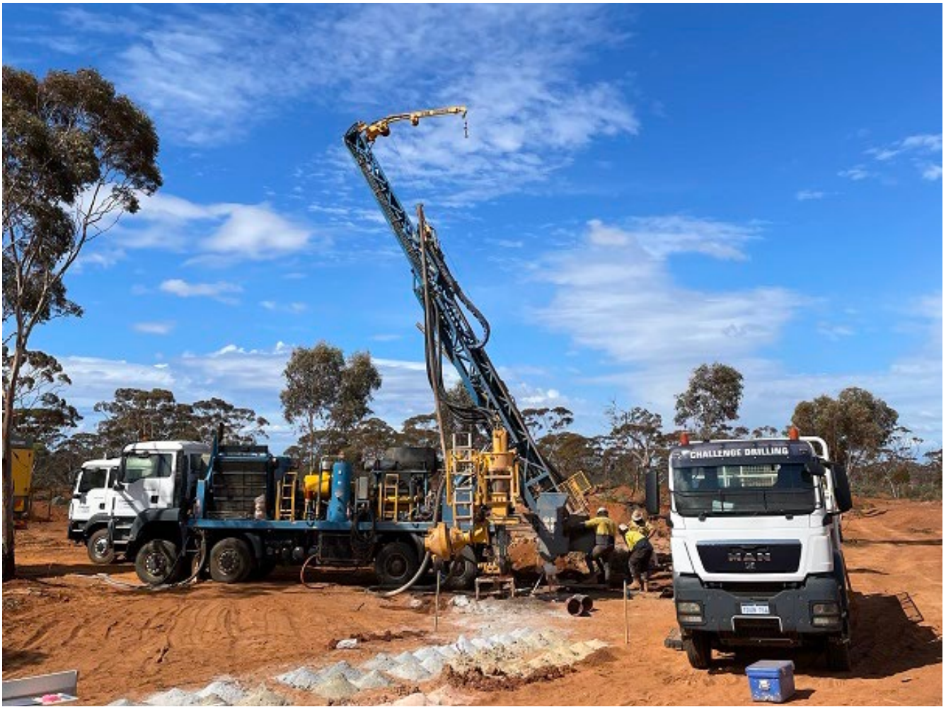
Image 1 – Theia In-Fill Drilling.
