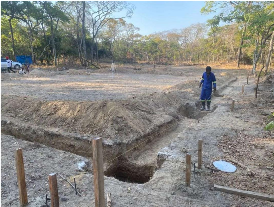
*Figure 12: Foundations being completed for core processing facility at Mumbezhi Project*
