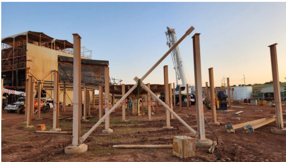
Photo 3: Boonanarring - Slimes Thickener dismantling
