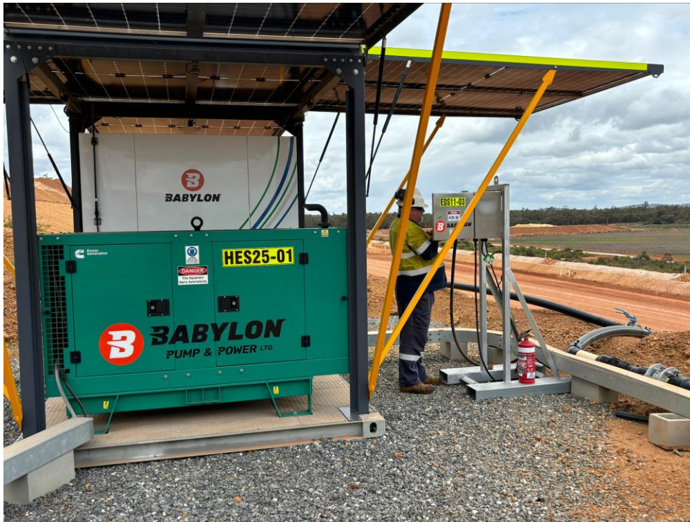
A recently installed hybrid power unit at a West Australian gold mine
