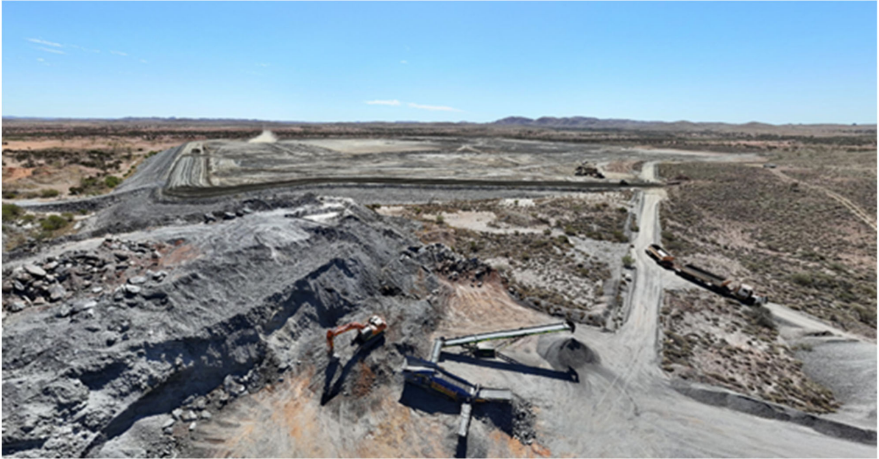
Figure 7: Showing the ongoing construction of lift #8 on the tailing storage facility.
