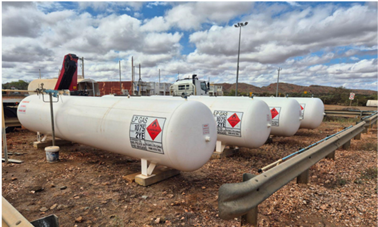
Figure 6: New LPG bullets have been installed and filled with gas for commissioning.
