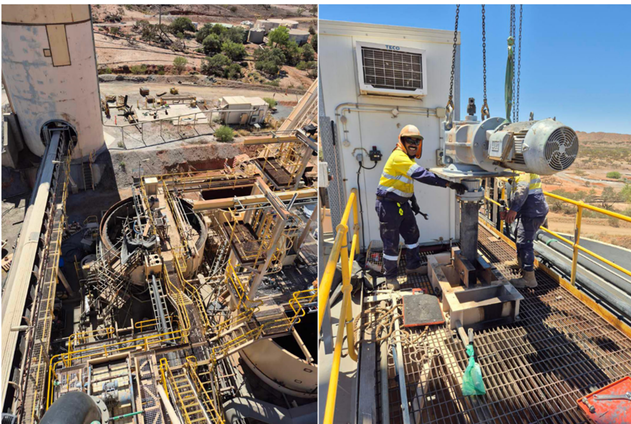
Figure 4: View of thickener and CIL infrastructure progress and MACA personnel installing an agitator shaft with new blades into position.
