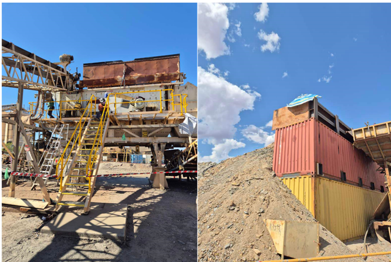
Figure 2: Showing the complete ROM wall and new walkways on the crusher screen.
