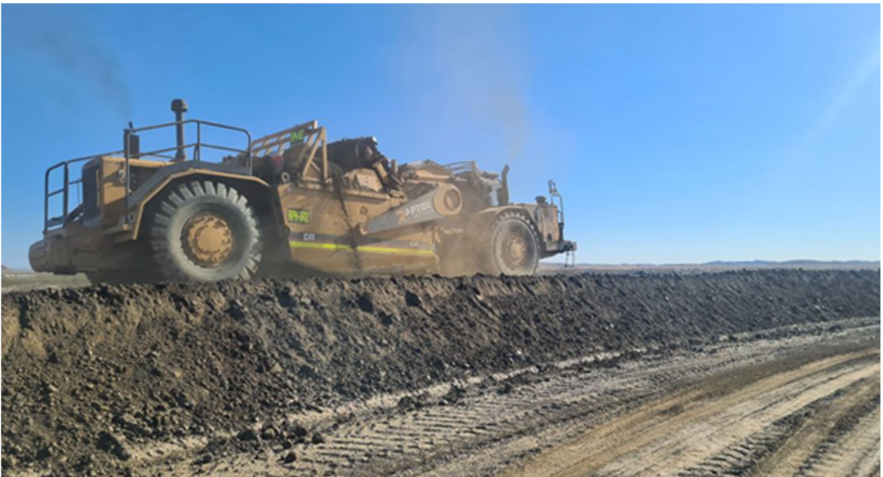
Figure 8: Showing scraper working on the tailing storage facility wall lift #8.
