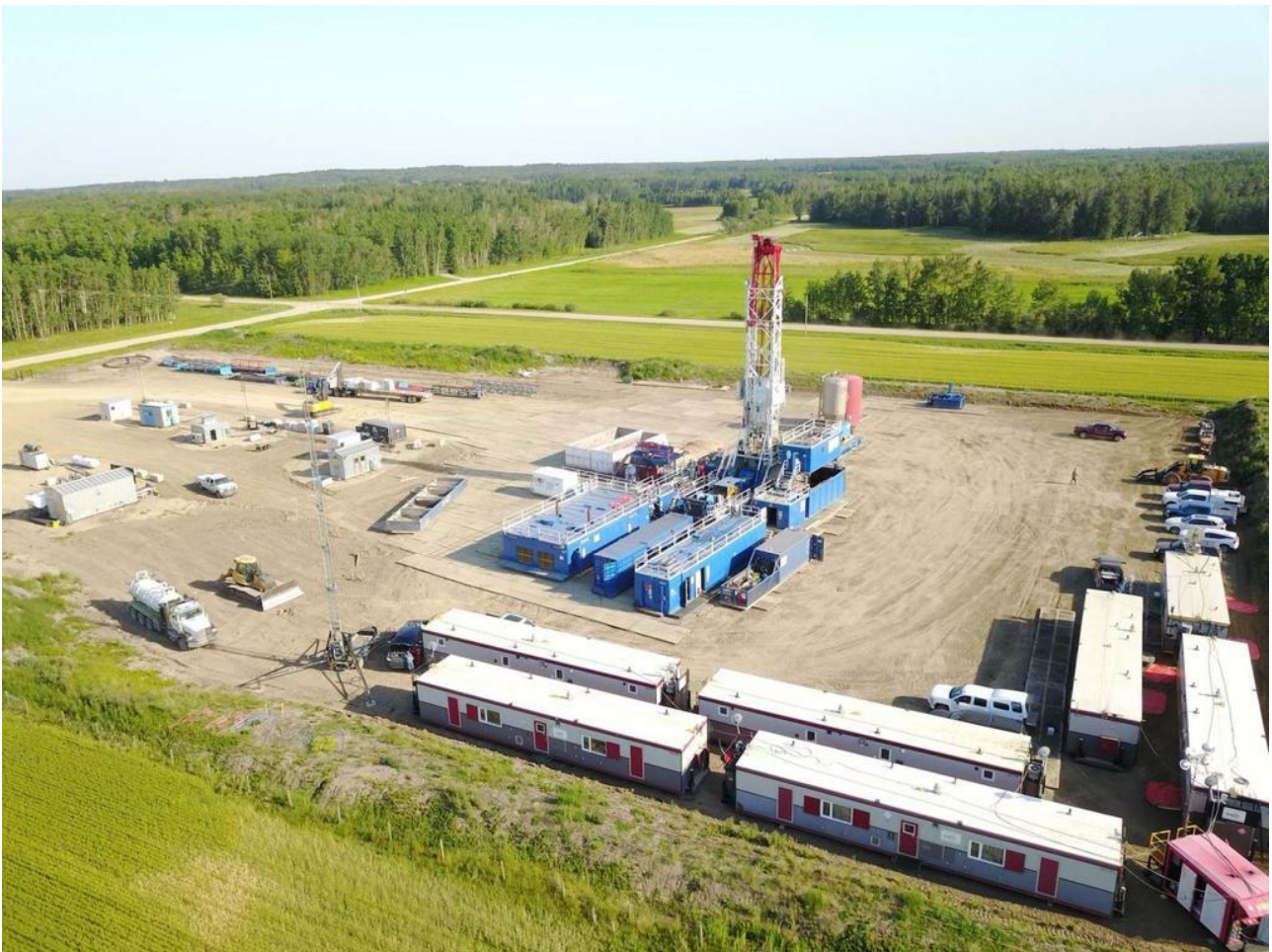
Figure 4 - Drill rig on site at Rex-4
